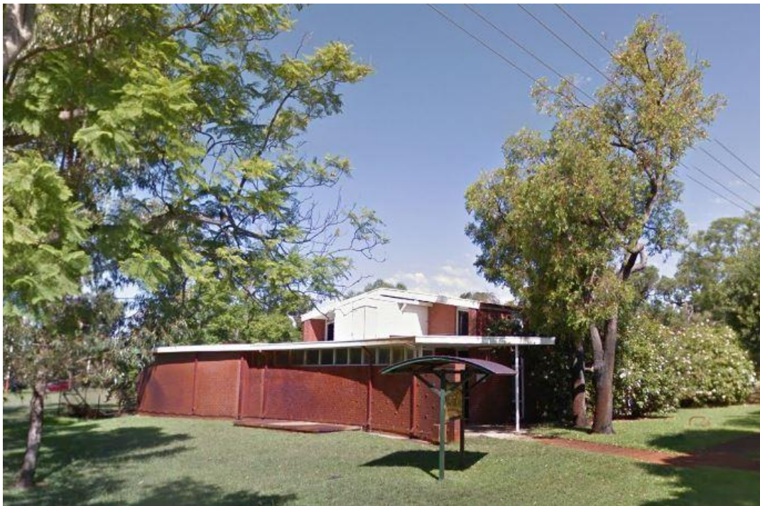
Hackett Hall in Draper Street Floreat was opened in 1960 (Google 2020).
